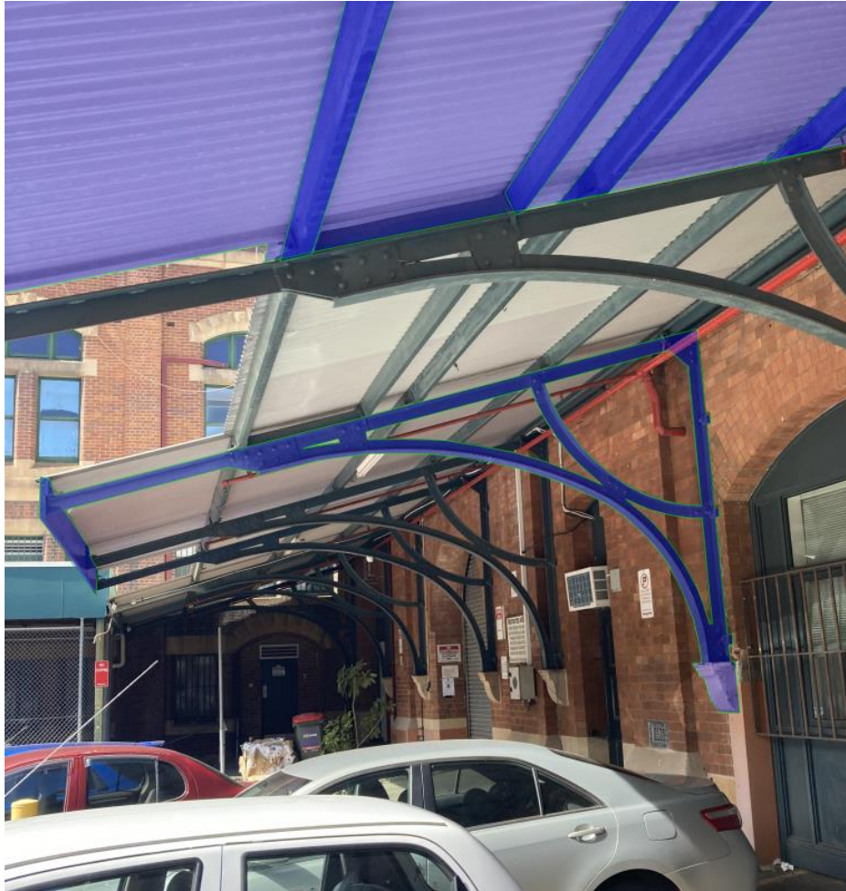
Figure 1-11: Southern awning structure
