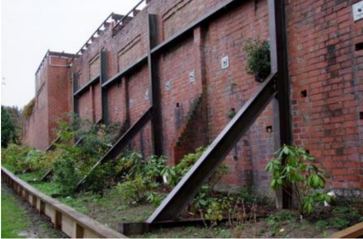
Figure 1-18: Heritage Wall Bracing Examples – Adina Hotel Side
