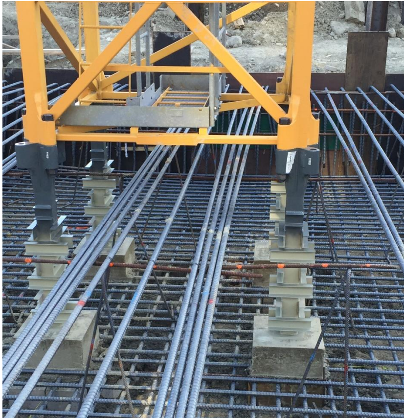
Figure 1-45: Tower Crane 2 Base
