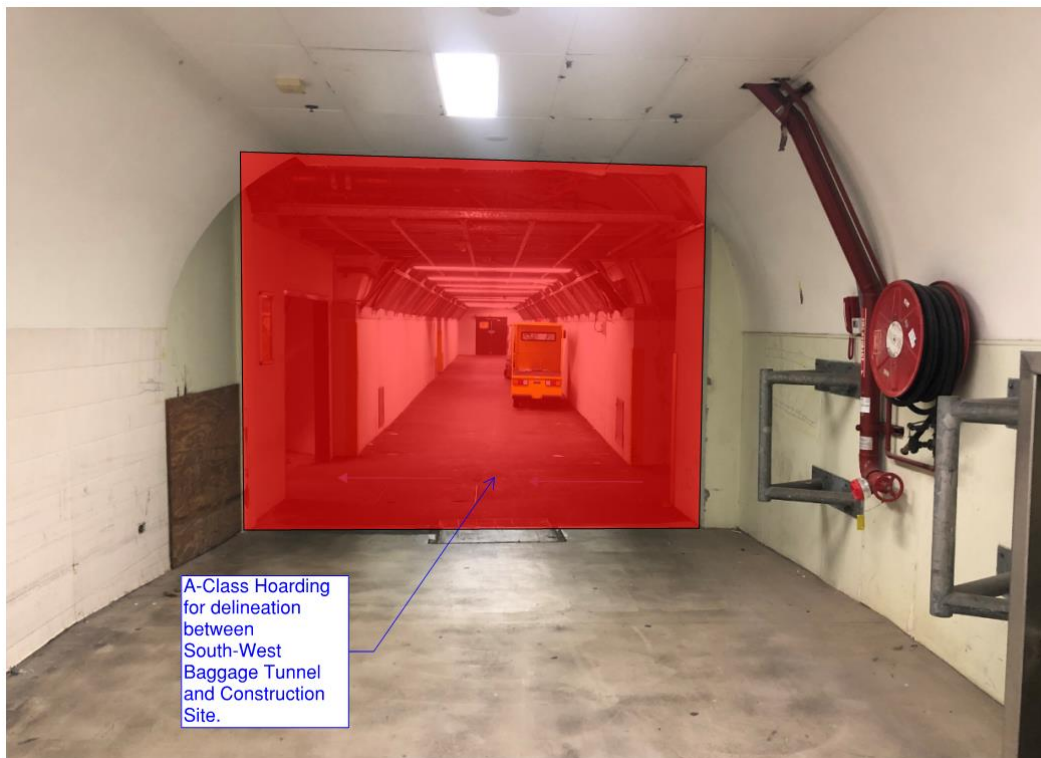
Figure 1-24: A-Class Hoarding – South-Western Baggage Terminal
