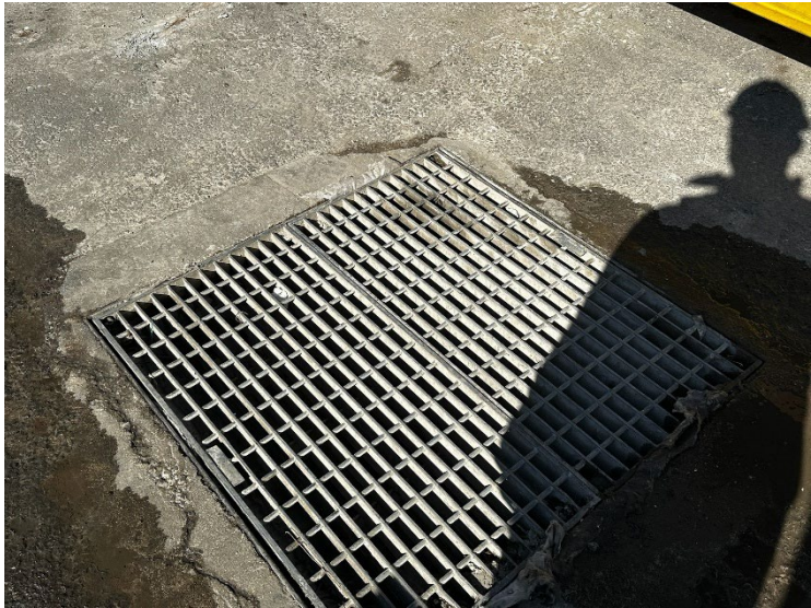
Photo 15: Drainage pit with pit protection
