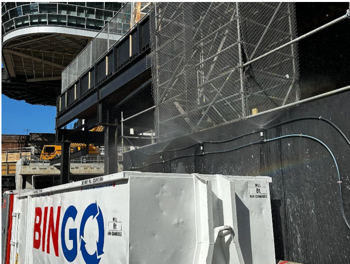
Photo 5: skip bin with water sprays for dust suppression
