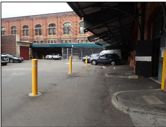
Figure 4.19 View south-east of Ambulance Avenue, showing the underside of awning over basement level.
