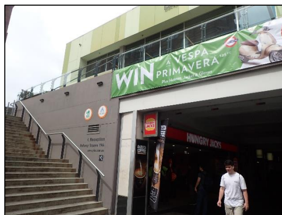
Figure 4.2 View north-east of stairs to YHA from Devonshire Street Tunnel.
