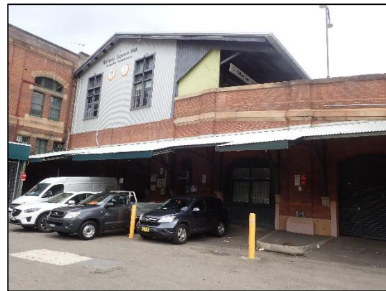
Figure 4.18 View south-east of level beneath the YHA.
