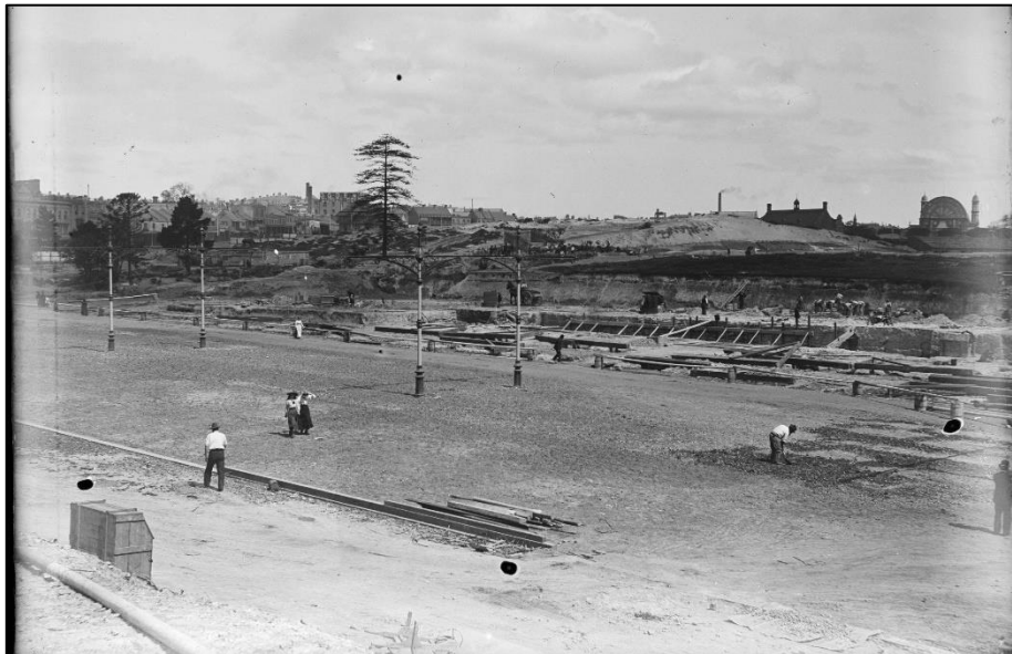
Figure 3.19 Eddy Avenue, levelled site with tramline stanchions in place, before paving. Looking south-east, cleared land for Central Station (Source: State Library of NSW, Box 14: Royal Australian Historical Society: photonegatives, ca. 1900-1925, IE8952327).
