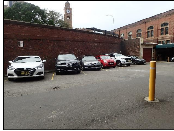
Figure 4.16 View north-east of retaining wall north of Ambulance Avenue. The Central Station clocktower is in background.
