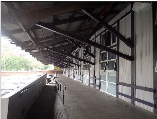
Figure 4.5 Western elevation of the YHA.
