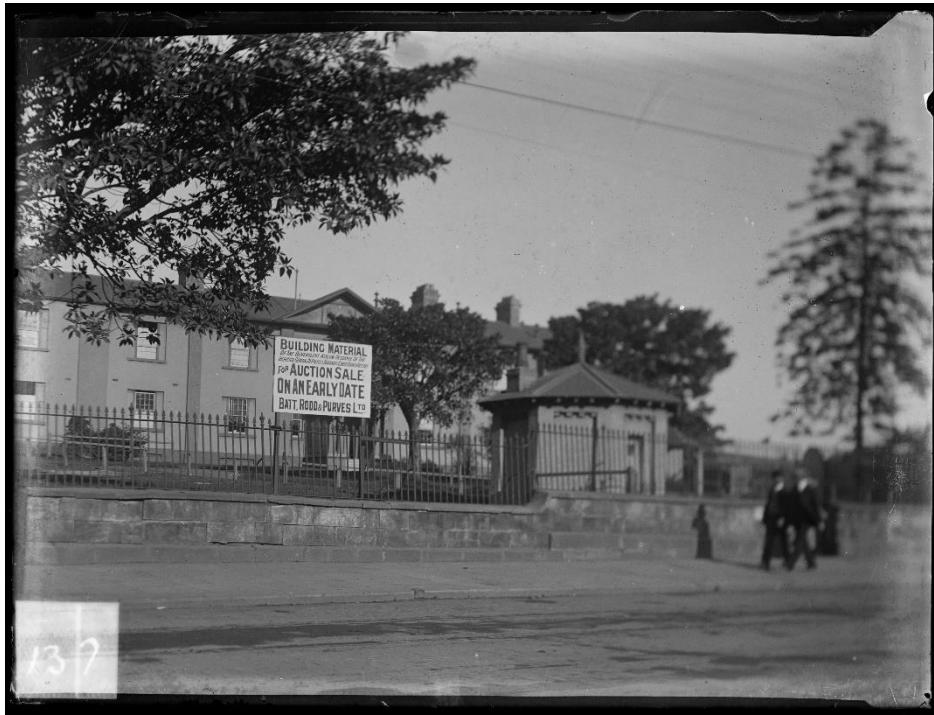
Figure 3.10 Benevolent Asylum on Pitt Street, sign for the auction of building material in forefront in preparation for the demolition and construction of Central Station. Note the slight uphill incline (Source: SL NSW, IE8546525, Glass Negatives of Sydney and Suburbs ca.1900-1914).
