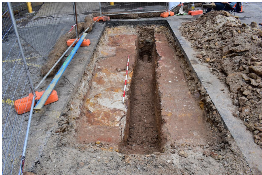
Figure 5.12: Service cut through the bedrock in Trench 2 (Artefact Heritage 2021).
