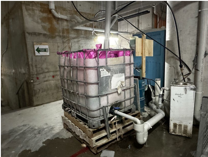
Photo 20: Innovative concrete washout capture system
