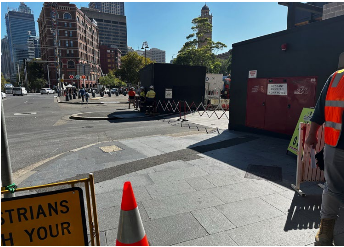
Photo 5: Supervised traffic and pedestrian control with operational boom gates
