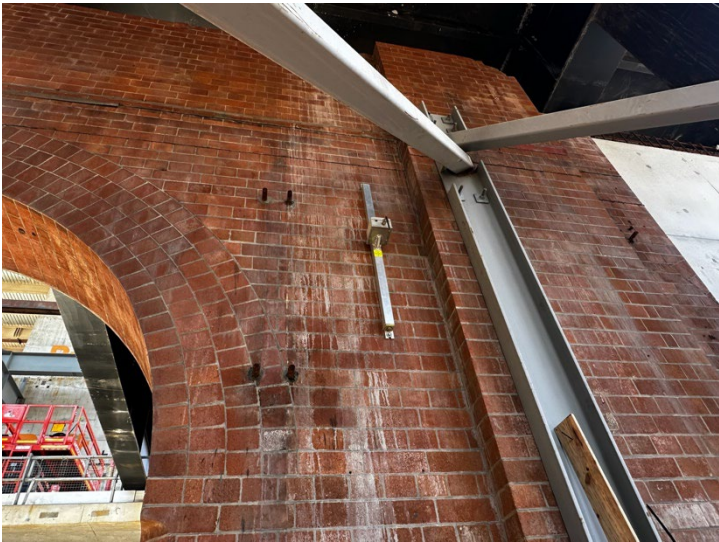
Photo 19: Heritage monitor and structural support
