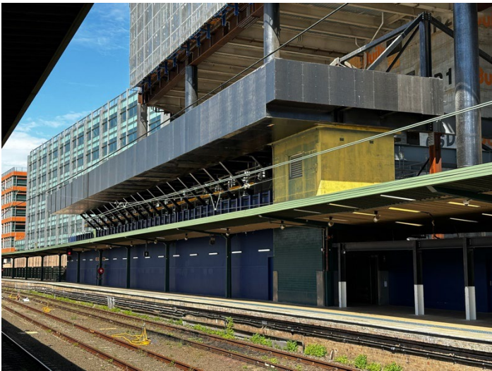
Photo 12: Catch protection hoarding over Central Station platform 1
