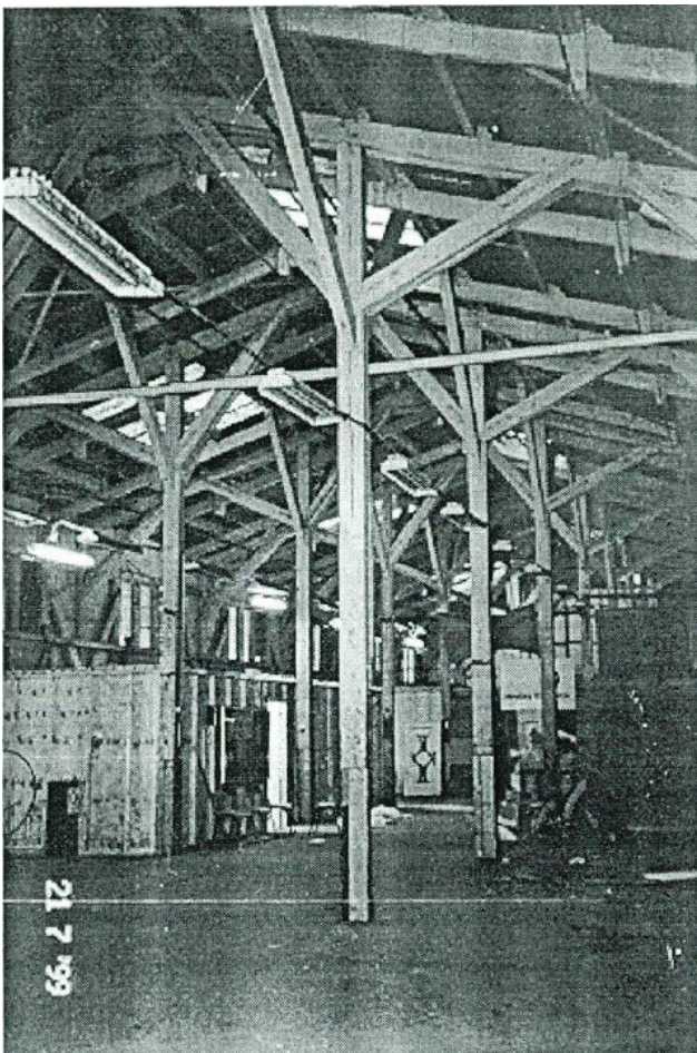
Figure 179 - The freestanding strutted timber posts that support the roof of the Inwards Parcels Shed.
