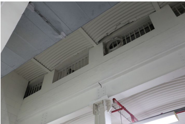
Figure 74 – Basement lights, with early bars and glazing still intact
