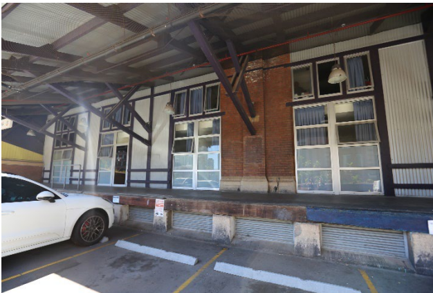
Figure 28 – Masonry piers on sandstone plinth at western elevation.
