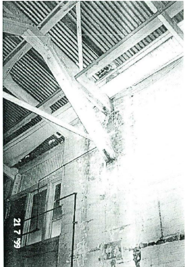
Figure 186 - Internally painted masonry pier and connection with roof framing.
