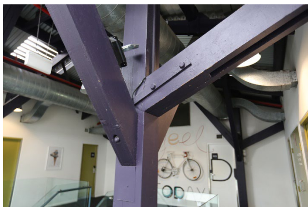
Figure 23 – Detail of timber post and struts
