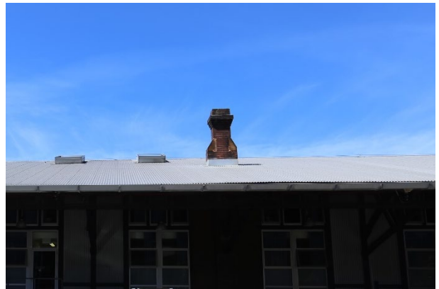
Figure 29 – Brick and sandstone corbelled chimney at west side of shed.
