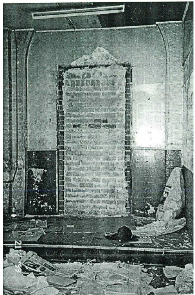
Figure 188 - East wall of the Inwards Parcels Shed at the junction with the southern end of the west wing of the Terminal building. The wall is rendered and the former opening was placed symmetrically with the archway.
