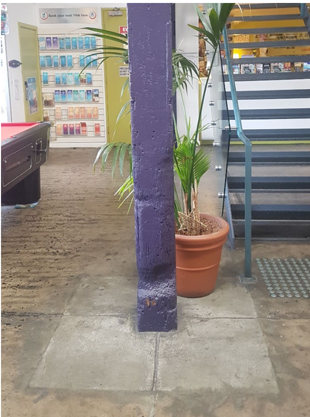
Figure 50 – Detail of timber column with signs of wear from original use
