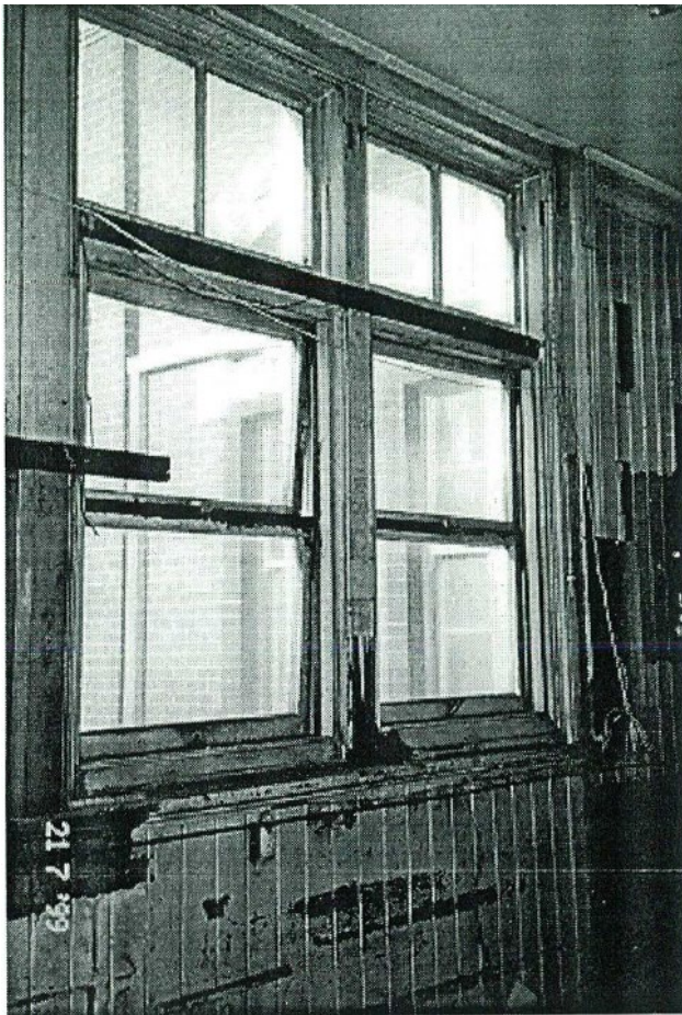
Figure 187 - North wall of Time Keeper's Office, internally lined with vertical timber boarding.
