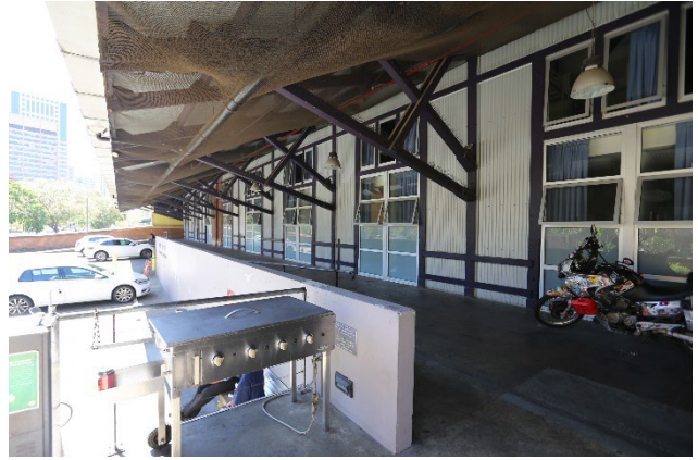
Figure 27 – West elevation of the shed, with the timber expressed frame and new aluminium windows
