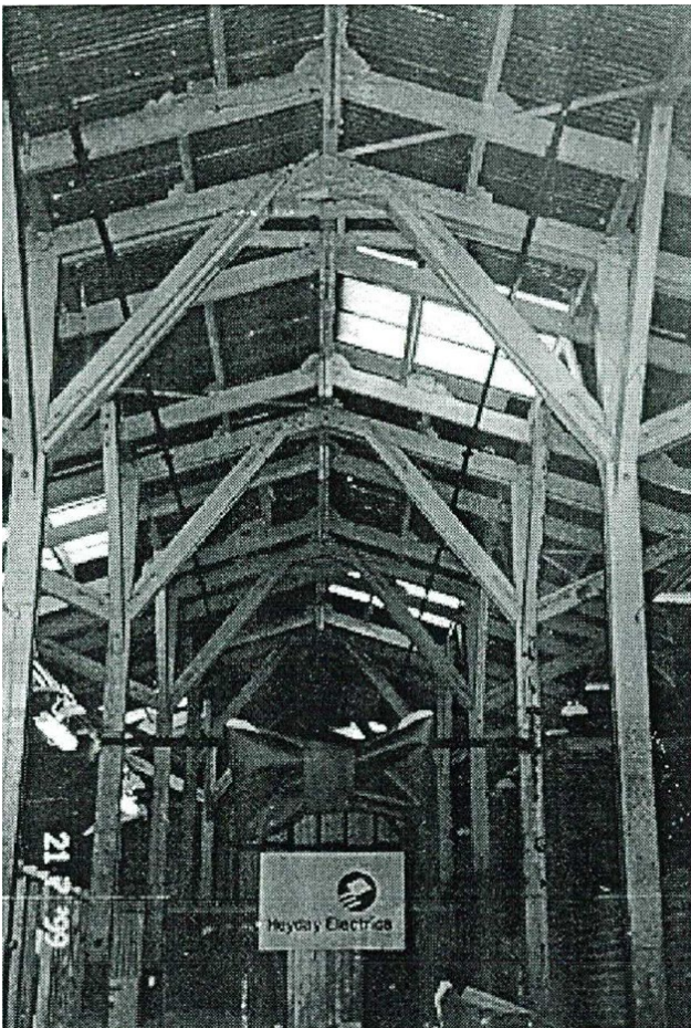
Figure 183 - Looking north within the central 'nave' created by the two rows of the freestanding struted timber posts.
