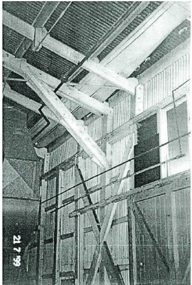
Figure 180 A strutted timber post incorporated into the wall structure of the Inwards Parcels Shed.
