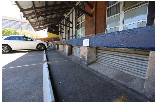
Figure 41 – Skylights under Loading dock and timber sleeper edging.
