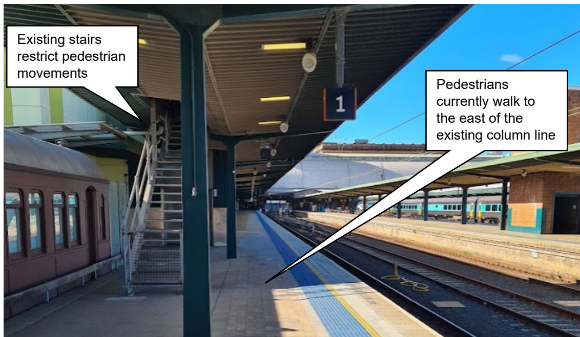
Figure 21 Central Station platform 1 (looking north)
